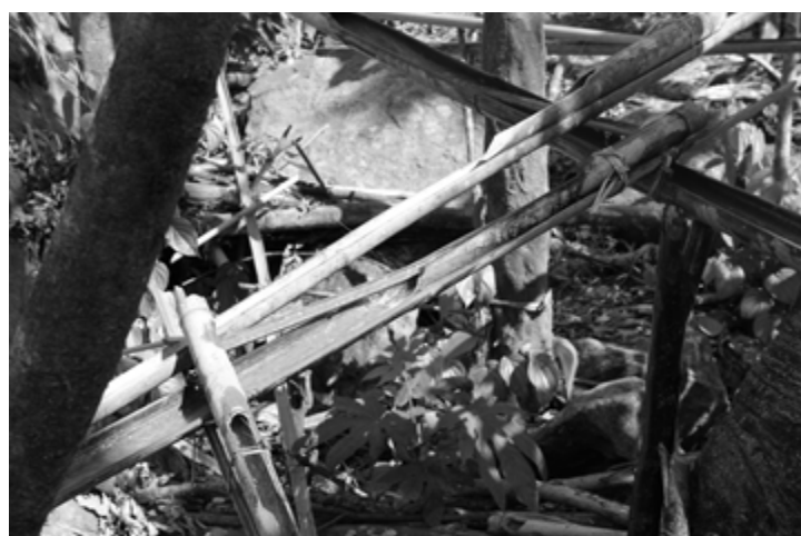
Plate No. 1: Bamboo networking for water distribution with regulators
